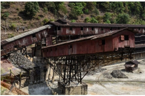
A refinery at the Bawdwin mine.
