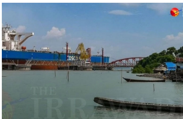
A crude oil tanker docks at Maday Island in Kyaukphyu Township in 2019.
