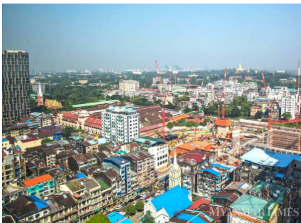
The Yoma Central development site in Yangon is seen in the distance.
