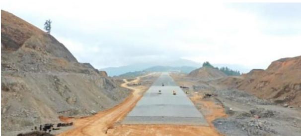
Construction site of the Surbung Airport in Chin State
