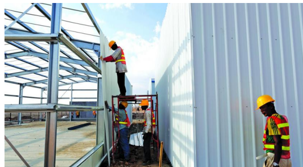
Construction work at the Thilawa SEZ
