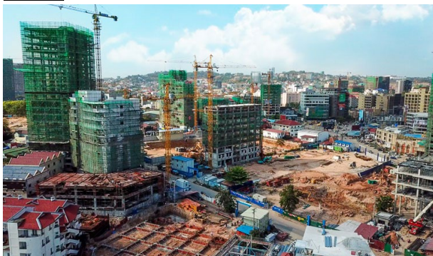
Aerial view of the under-construction buildings in Sihanoukville
