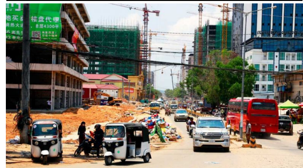
Construction in Sihanoukville
