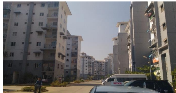
Low Cost Housing Project in South Dagon Township
